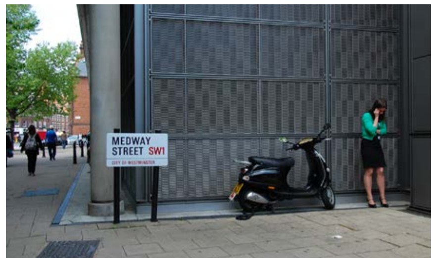
Closed frontage with grilles and servicing
