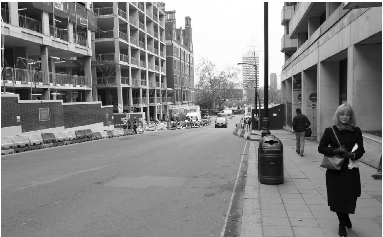
View south along Arundel Street towards Temple Station and the site of the proposed Garden Bridge
