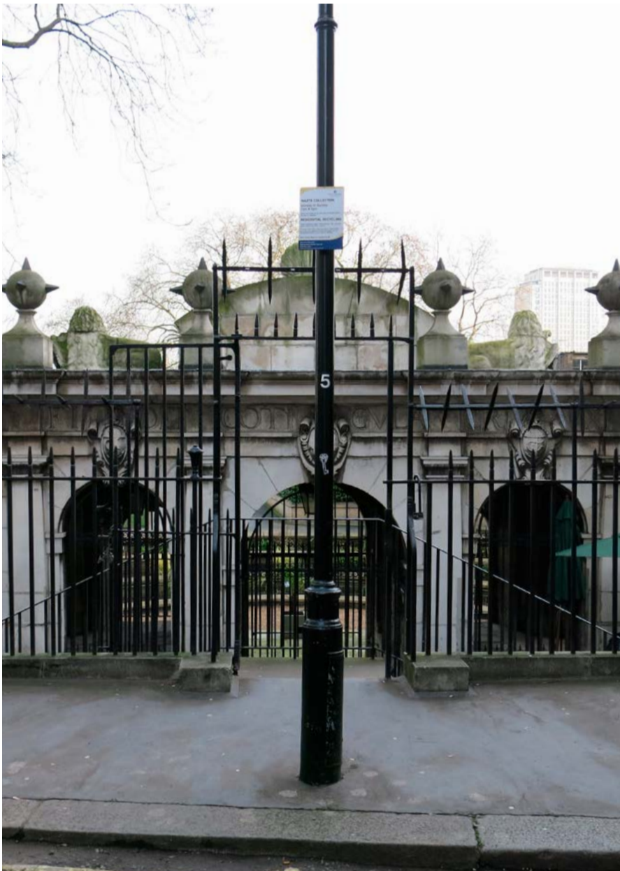
Gates and railings obscure the Grade I listed York Watergate, blocking views to the historic gateway to the river and making onward connections confusing for pedestrians
