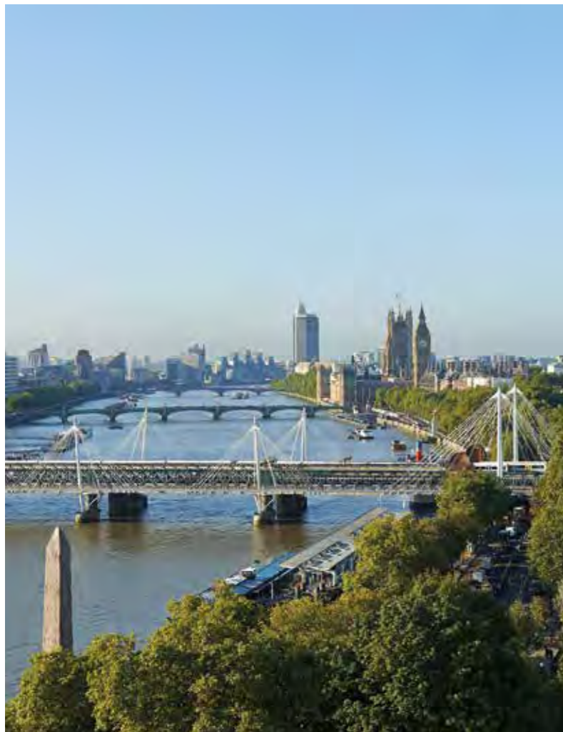
VICTORIA EMBANKMENT GARDENS
