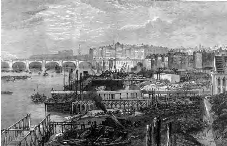
Above: Bazalgette's Embankment under construction in the 1870s. Below: Schematic section through the Embankment, showing cut and cover tube line and sewer locations, reclaimed from the river
