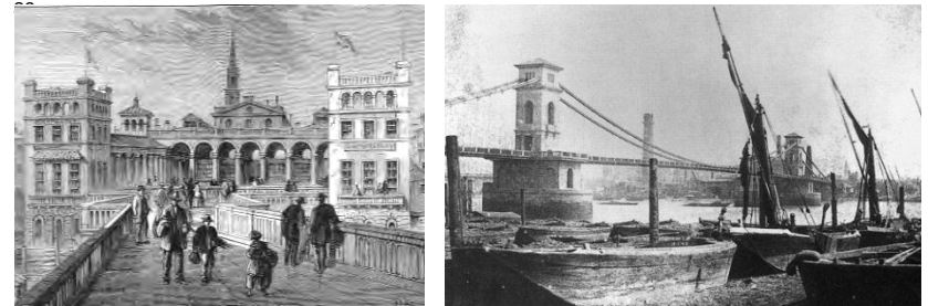
Above left: Hungerford market, c1850, approached from Hungerford Bridge Above right: Brunel's Hungerford Footbridge. Built in 1845 and replaced by the Charing Cross Railway Bridge in the 1860s, using the same buttresses.
