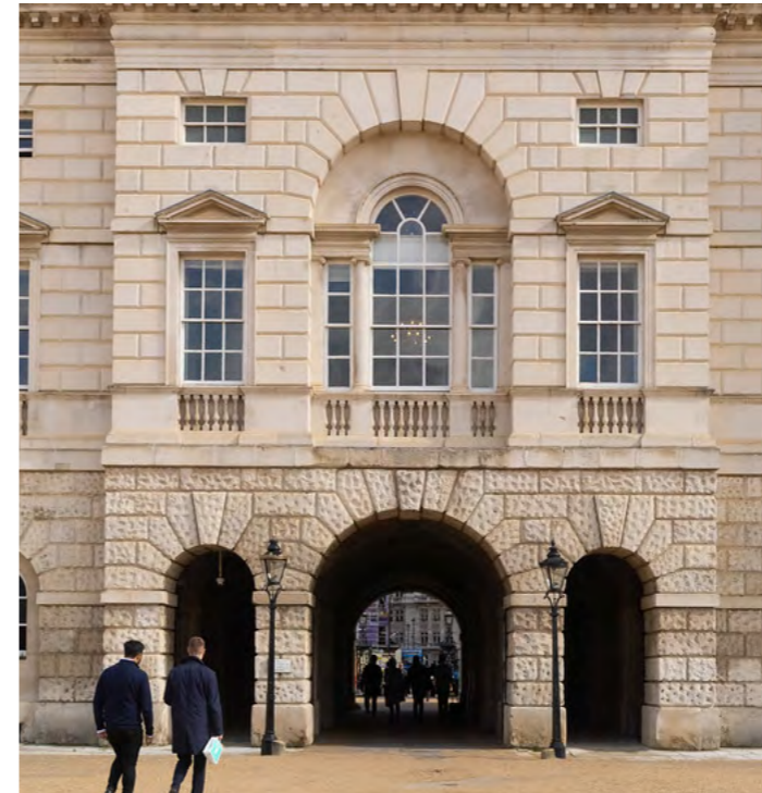
Fig. 108 - Pedestrian access from Horse Guards Road to Whitehall via Horse Guards Parade
