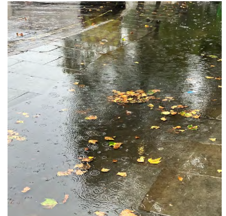
Fig. 269 - Flooding issues on the corner of Whitehall Place and Northumberland Avenue
