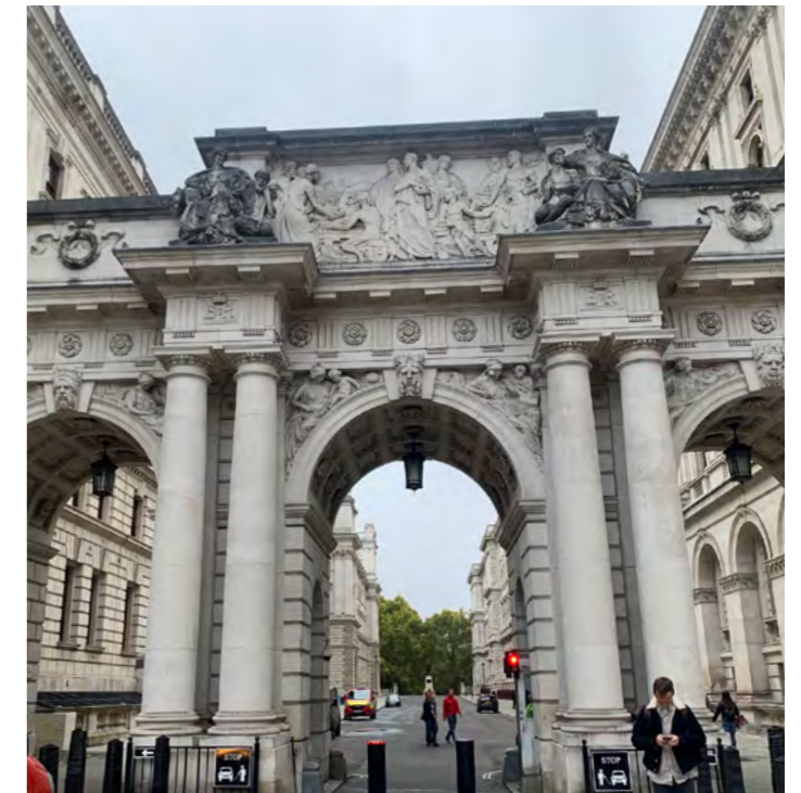
Fig. 161 - Bollards to control vehicle access to King Charles Street
