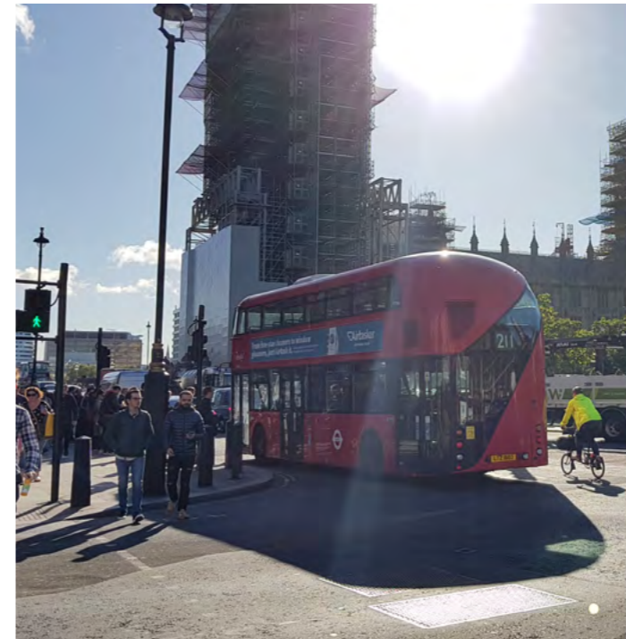
Fig. 212 - Bridge Street looking towards the Elizabeth Tower
